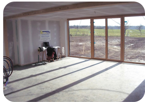
South-exposed bay window: significant solar supplies in winter
