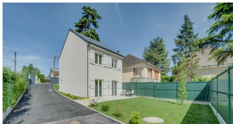
Figure 1: Maison Ermont - Ecolocost
